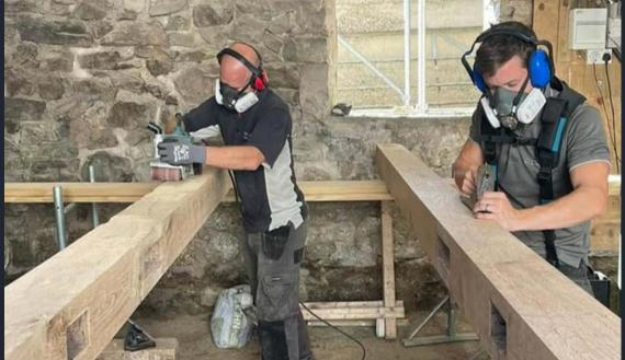
At Bynbuild, we undertake a range of listed building works throughout the Chesire and North Wales area. Recently we delivered works to a Grade 2\* listed building, replacing a traditional structural H Frame using hand tools to make traditional mortise & tenon biscuit joints
