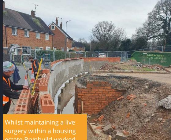
whilst maintaining a live surgery within a housing estate Brynbuild worked with engineers to come up with a solution to build a substantial wall to replace a defective 70m wall involving road and pavement closures for the NHS.
