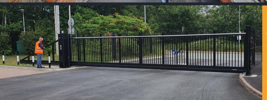
Brynbuild installed new industrial automatic gate and perimeter fencing to the whole Tate& Lyle site in Mold. Site constraints included utilities mains coming in under the new entrance whilst manageing zero strike rate.
